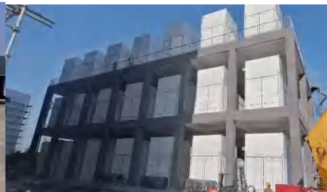
Sound-absorbing package (Super silent solution)
