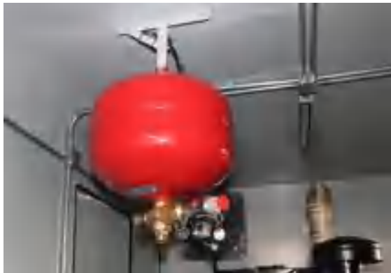
Heptafluoropropane fire extinguish system
